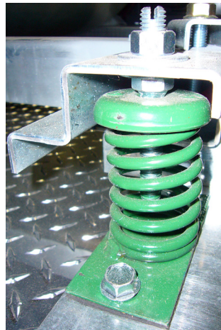
Figure 8: Spring Isolation
